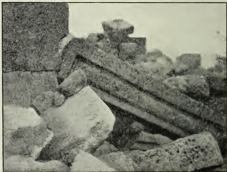
FIG. 274.—Hayyat, lintel of door between narthex and nave.
